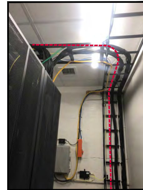
① DATA ROOM: TRANSITION CABLE FROM EXISTING HDPE CONDUIT TO DATA RACK CABINET. PULL CABLE THROUGH EXISTING HDPE CONDUIT AND ROUTE WITH EXISTING CABLE TO CABLE TRAY AND RACK LOCATION. LEAVE 25' COIL FOR SPLICER. 1ST RACK FROM THE SOUTH
