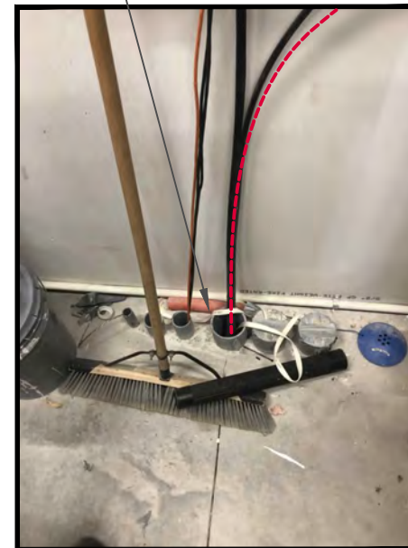
② MECHANICAL ROOM: TRANSITION CABLE FROM EXISTING HDPE CONDUIT TO HDPE CONDUIT ROUTING TO DATA ROOM. PULL CABLE THROUGH EXISTING HDPE CONDUIT AND ROUTE WITH EXISTING CABLE TO DATA ROOM ENTRY CONDUIT ON WEST WALL.
