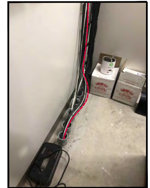
① DATA ROOM: TRANSITION CABLE FROM EXISTING HDPE CONDUIT TO DATA RACK CABINET. PULL CABLE THROUGH EXISTING HDPE CONDUIT AND ROUTE WITH EXISTING CABLE TO CABLE TRAY AND RACK LOCATION. LEAVE 25' COIL FOR SPLICER. 1ST RACK FROM THE SOUTH
